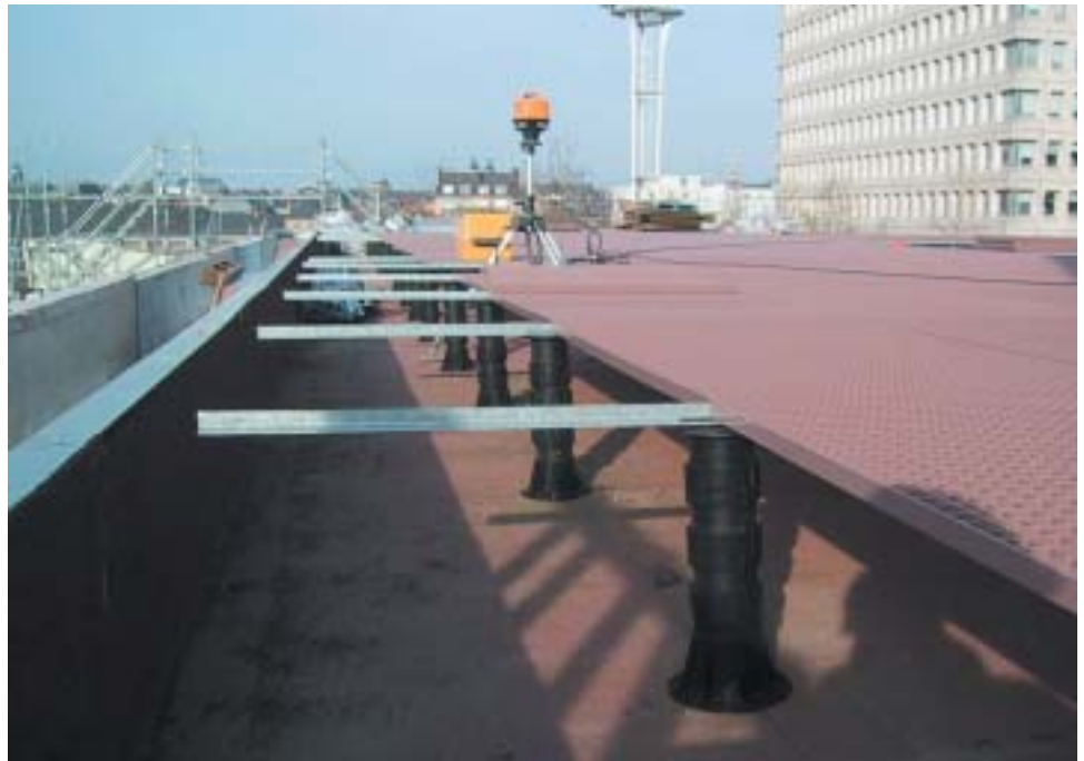
By adding special couplers heights of up to 60 cm can be reached
