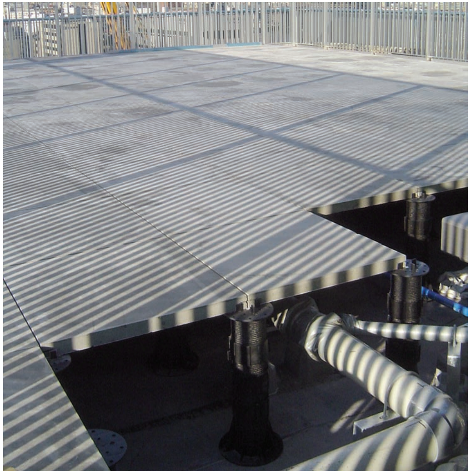
Canal Court Public Housing project in Tokyo, Japan: tiles 600 x 600 x 60 mm, covered heights from 240 to 600 mm, over a total area of 3000 sq m.
