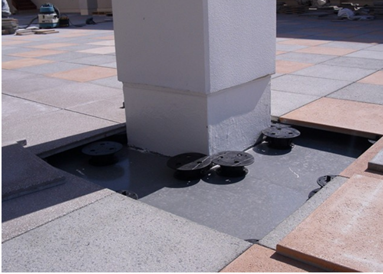
Fixing of stone tiles on Buzon pedestals around a pillar is no problem.
